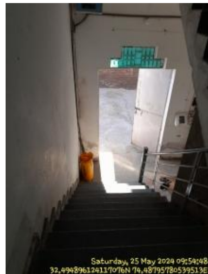
Missing Handrails.jpg
